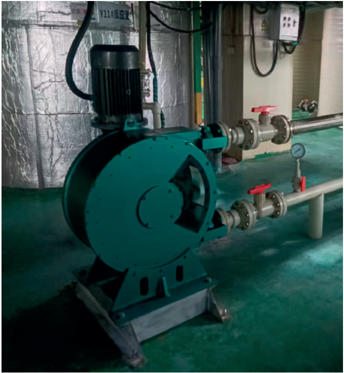
06 ▶ Magnetic material pumping
